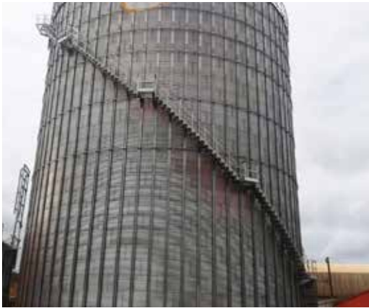
— Photo of spiral stairway on mod. FP flat bottom silo with platform in compliance with european standards
