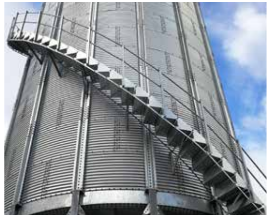
— Photo of spiral stairway with safety handrail
