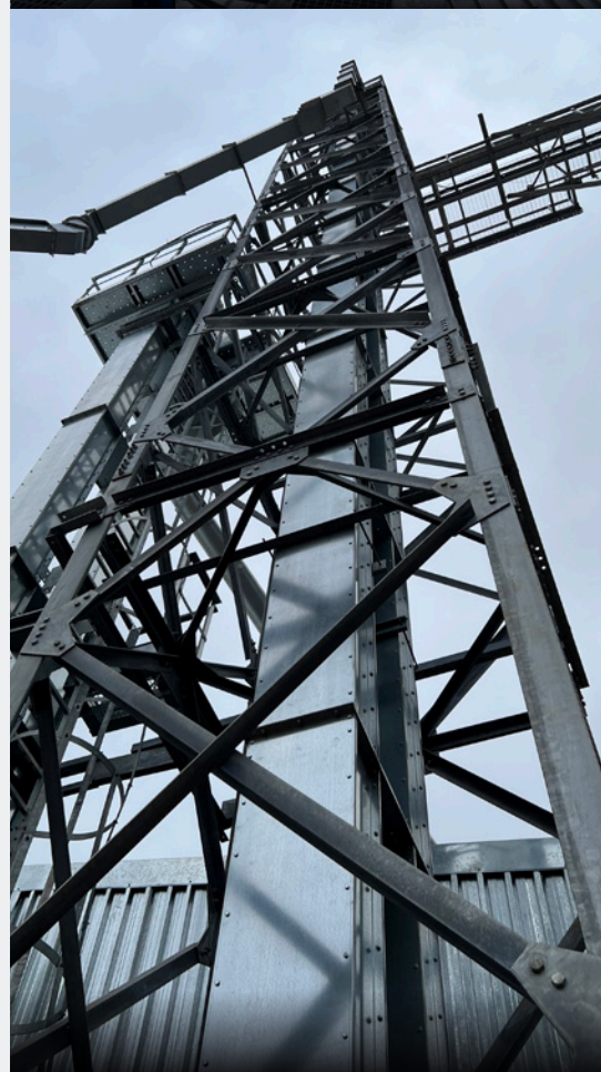
Catwalk type B - with double walkway
